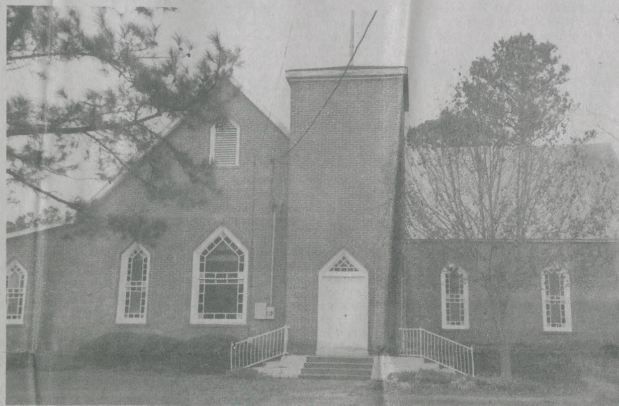
WEST HILL STREET FIRST BAPTIST CHURCH IN WARSAW is a historical treasure. Founded by freed slaves in 1867, shortly after the Civil War, it was first called Bear Swamp Baptist Church and located three miles east of Bowdens. The present building was erected in 1882 after members had worshiped for years using tree branches and brush for shade with benches made of mill scraps. Christmas in Warsaw will begin at this historic church with a song service from 2:00 to 2:30 p. m. on Sunday, December 5. (Photo Jo C. Jones)
