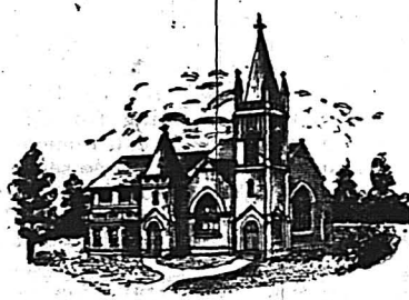
Baptist House of Worship, Waynesville, N. C., in process of construction.
