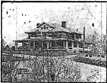
A Children's Home Building, Winston-Salem, N. C.
