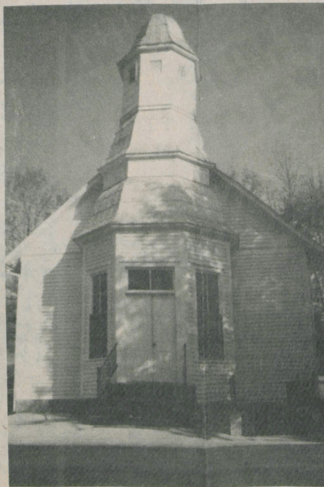
SPEEDWELL BAPTIST CHURCH OBSERVED ITS 85th anniversary Sunday. The existing church building was constructed in 1913-14. The church's current membership totals 241.
