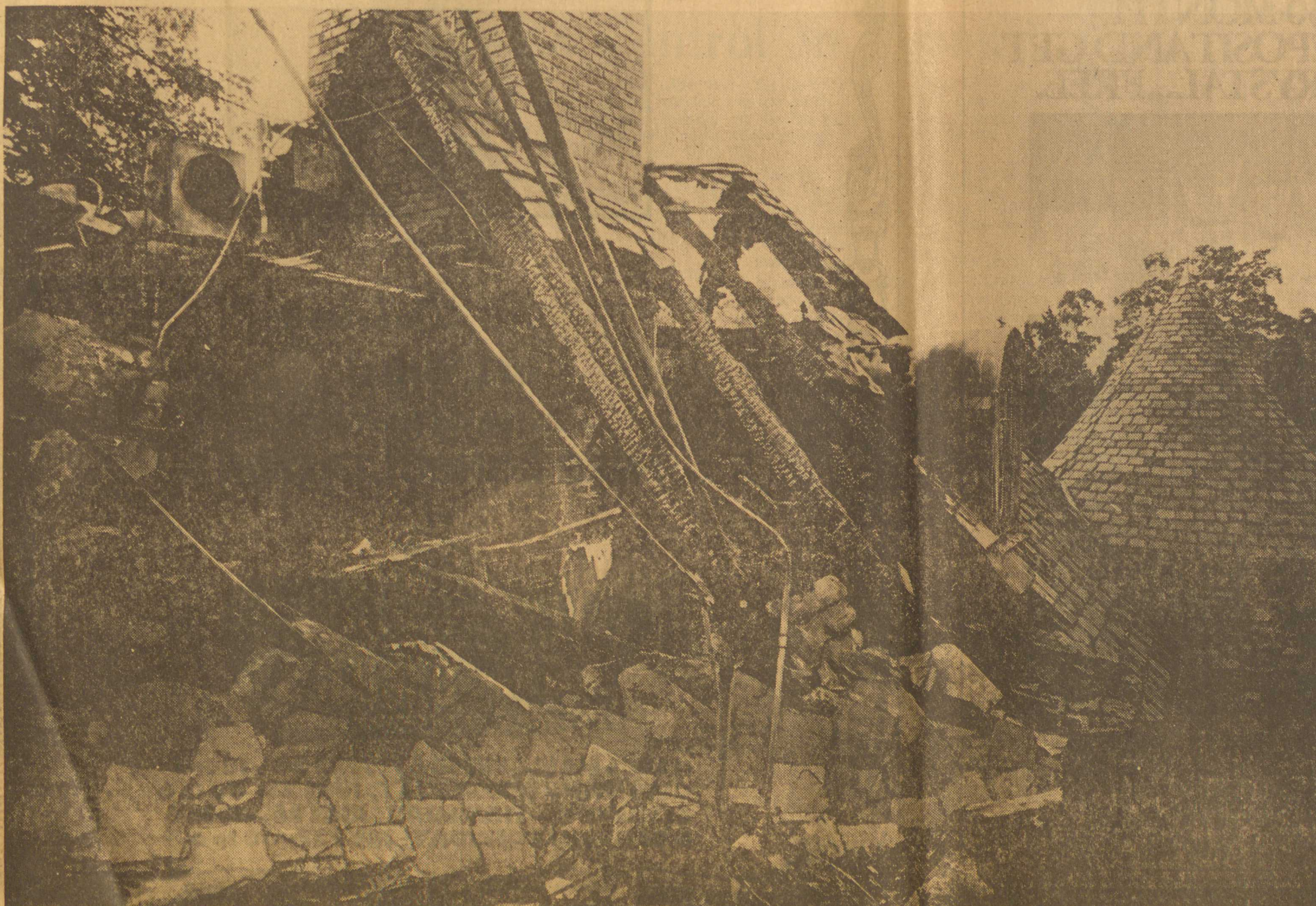
Though the roof collapsed, this section of the attic was strong enough to hold the rubble.
