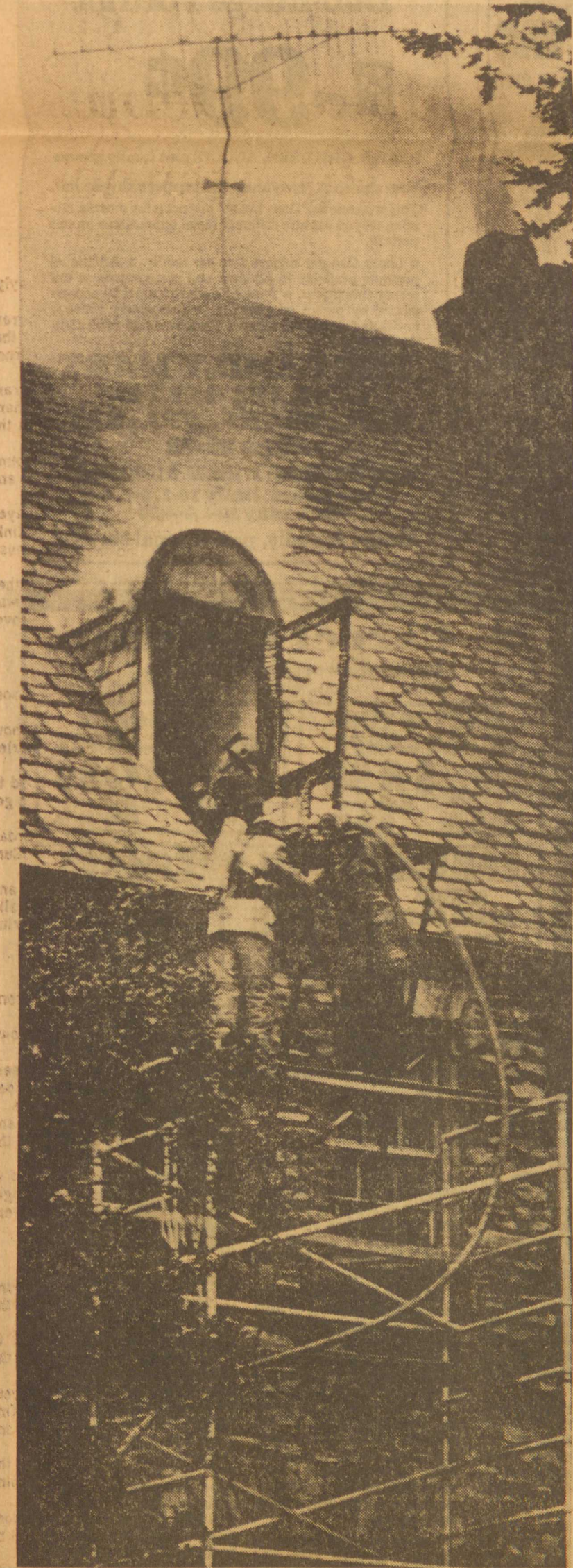
This window is where the smoke first appeared in the fire Sunday night.
