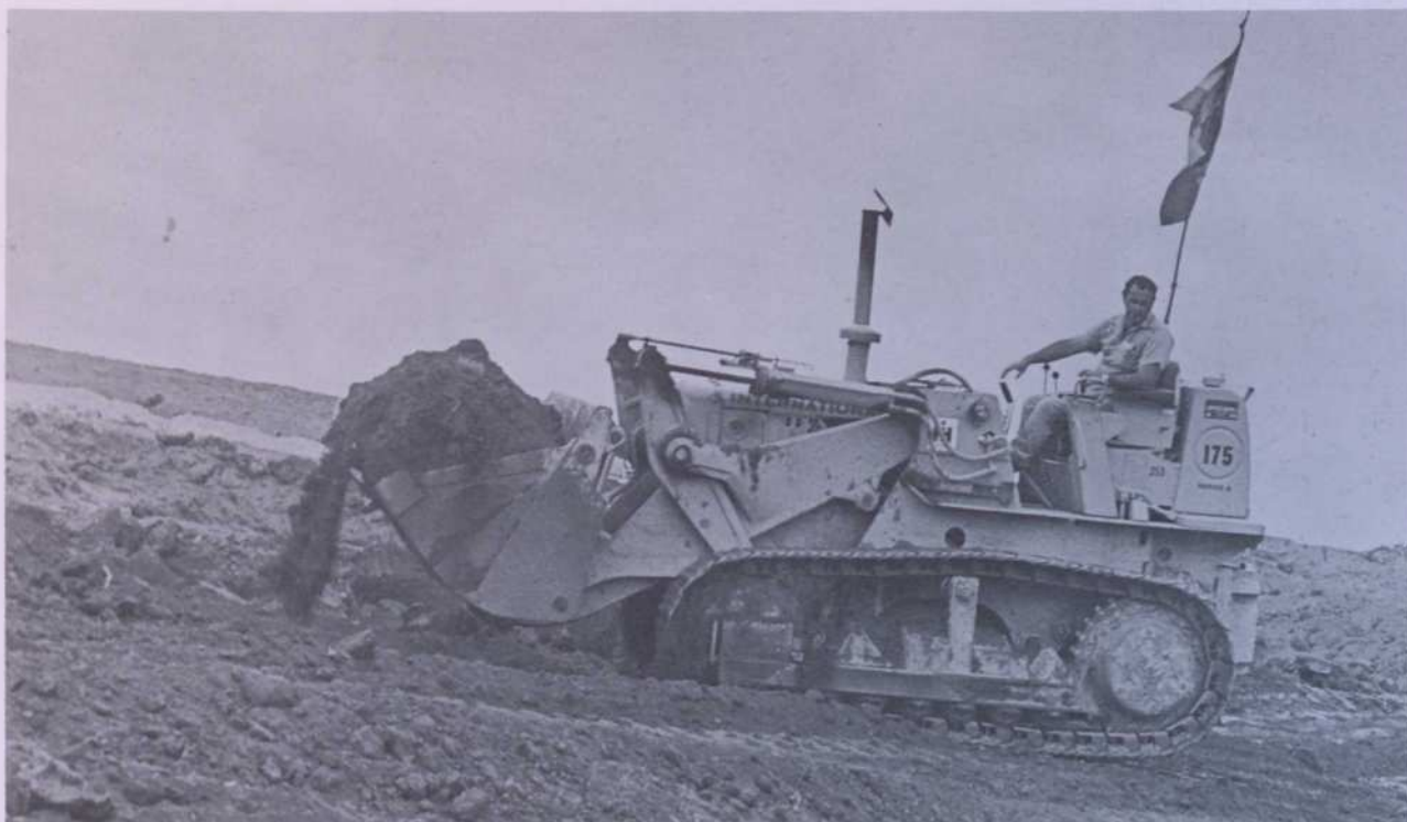
International 175B Loader on grading job in Piedmont North Carolina. The Loader is owned by L. A. Reynolds Company at Winston-Salem.
